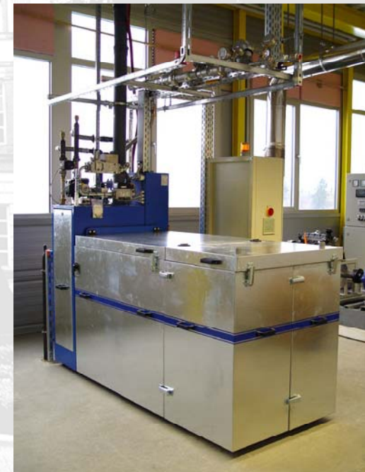
Biogas engine-cogeneration unit
