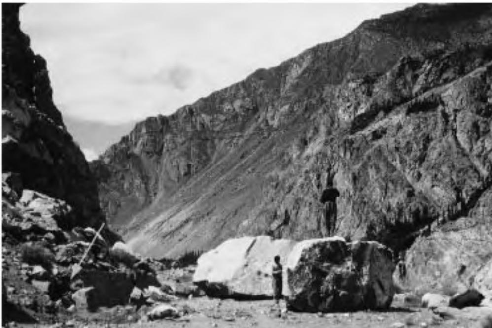
↑ *Photo 22.* Large-sized rockfall event in gneiss bedrock close to Sarat (2300 m) in the Hunza valley. The boulder with a diameter of 2 m left the roadway of the Karakoram Highway almost intact. The adjacent stone wall has been destroyed by debris slides (✓). The roadway shows a hole (▼) which was caused by the boulder at the back. (Photo L. Iturrizaga, 16 September 1992.)
