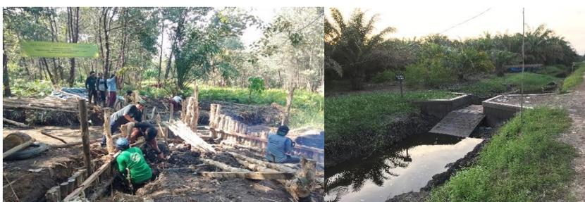
Figure 5 Building of a canal block to retain soil moisture in Seponjen, Jambi Province. Picture taken by the Author 2019
