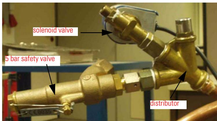
**Figure 2-49.** Valves and Distributor for Liquid Nitrogen (Side View)
