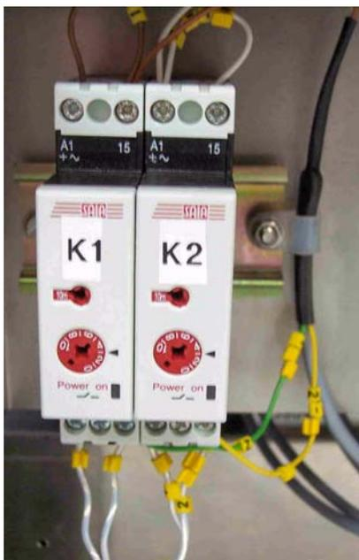
**Figure 2-10.** Safety Switch-Off for Acid Valve
