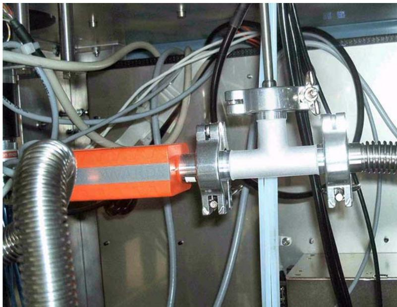
**Figure 2-14.** Position of VM2 Fore Vacuum Gauge
